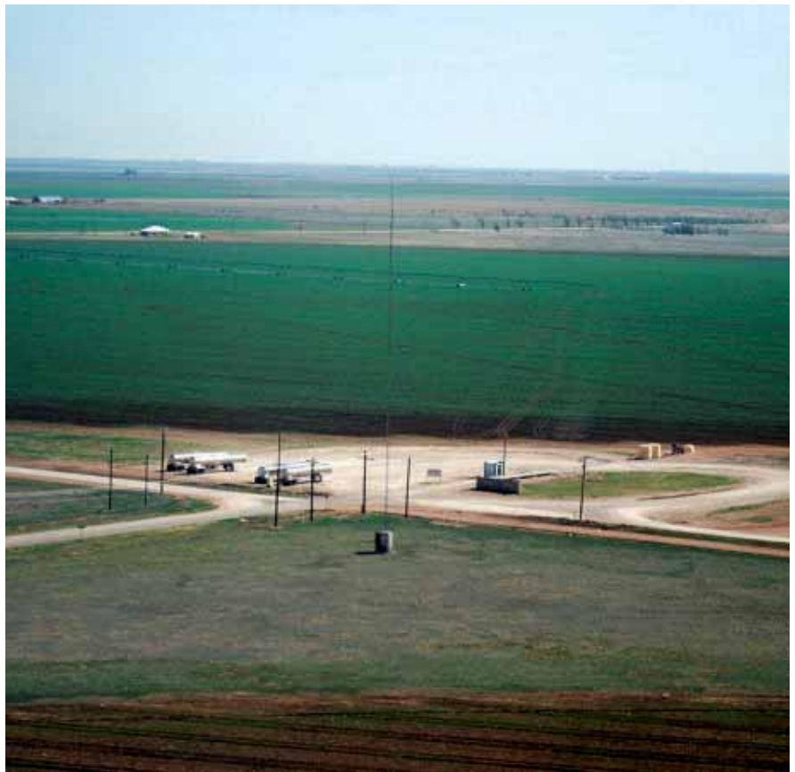
An aerial view of a real time kinematic (RTK) tower illustrates the diminished visibility of the tower for low-level aviation given certain atmospheric conditions in conjunction with power lines and various other distractions on the perimeter of the field. As Perry Hofer demonstrated, aerial applicators can work toward safer tower siting, marking and lighting by making their case before local Planning and Zoning Commissions on the effect of towers on aviation safety.
