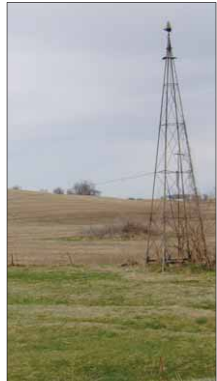
Figure 4. All man-made obstacles in fields must be investigated; this one has an unexpected wire running to it. Expect the unexpected!
