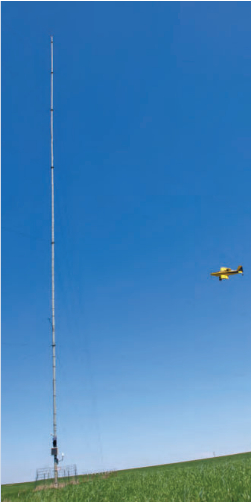
Under a new law in South Dakota, the upper third of this tower would need to be painted orange and white to help make it “recognizable in clear air during daylight hours.”
